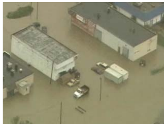
Figure 2-8 – Madison Avenue Business Flooding
